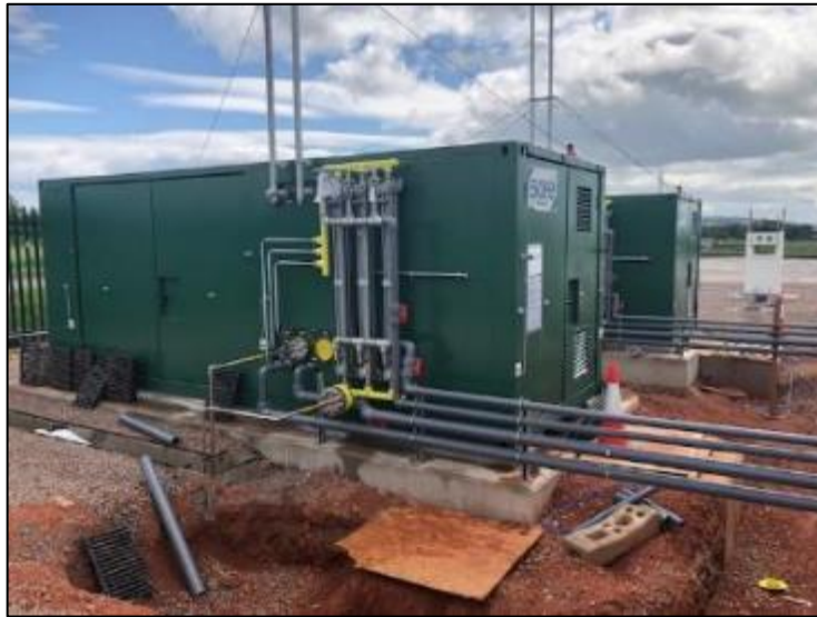
Compressor during installation
